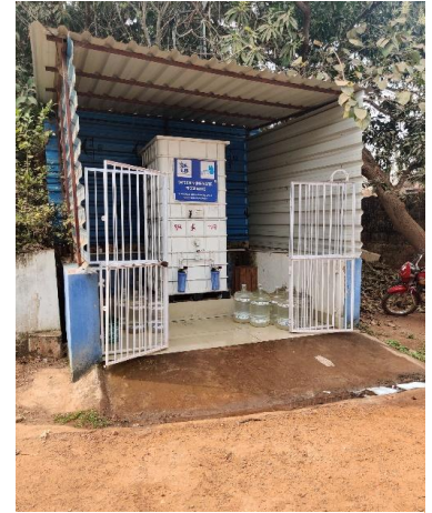
Water Purification Structure in Khorda
