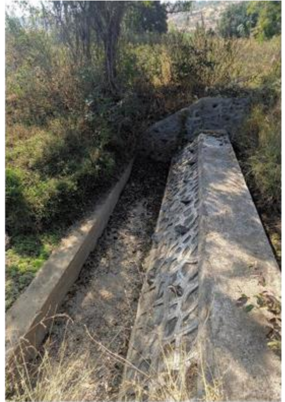
Earthen bund built in Aurangabad
